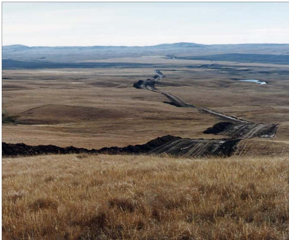
Pipeline Construction Through Rough Fescue Grasslands, Photo Courtesy of Jane Lancaster, Kestrel Research Inc.
